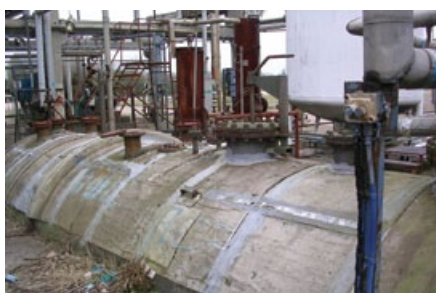
Figure 12 Lagging on large petrochemical vessel
