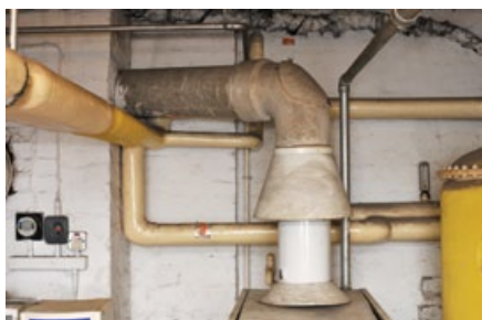
Figure 34 Asbestos cement boiler flue
