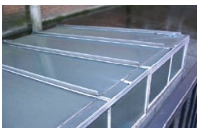
Figure 31 Chrysotile string on skylights
